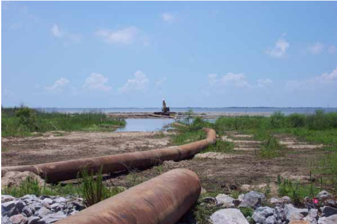
Photo 14. Discharge pipe across dike, pasture land, and existing wetlands
