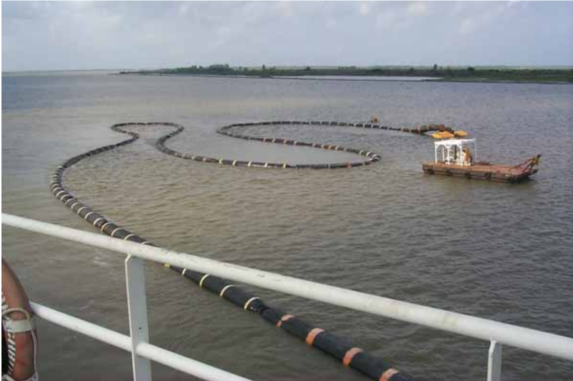
Photo 13. Anchor barge (skidder) holding floating hose
