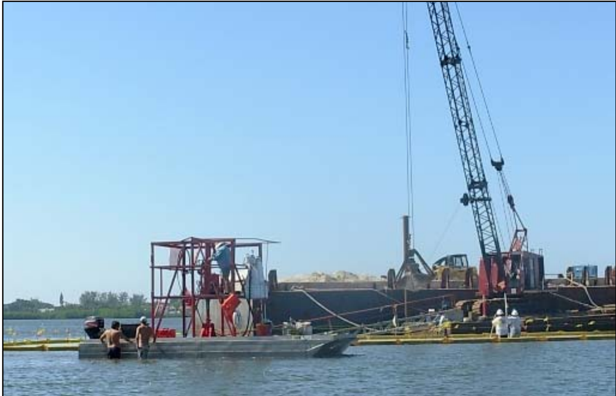
Figure 4. GUTS salvages seagrass near dredging operations in Florida. (Photo by Seagrass Recovery, Inc.)
