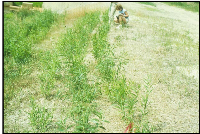
Figure 1. Willow stake plantings (photo provided by Sotir & Associates)
