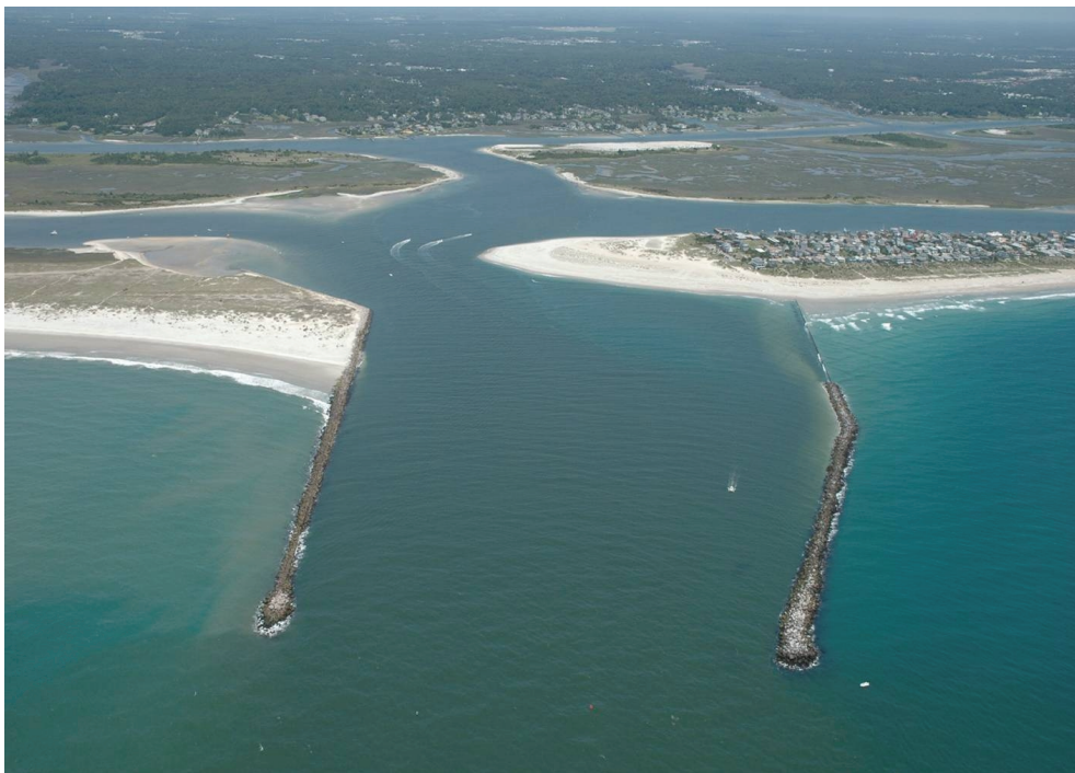
Figure 3. Stabilized inlet, where jetties impede sand flow parallel to the barrier beach, reducing potential for formation of ebb and flow sandbars and sandspits. Photo by Walker Golder, National Audubon Society.
